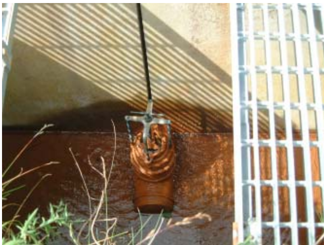
Figure 5.26.5. Outflow structure – there are two of these valve regulators for each cell.
