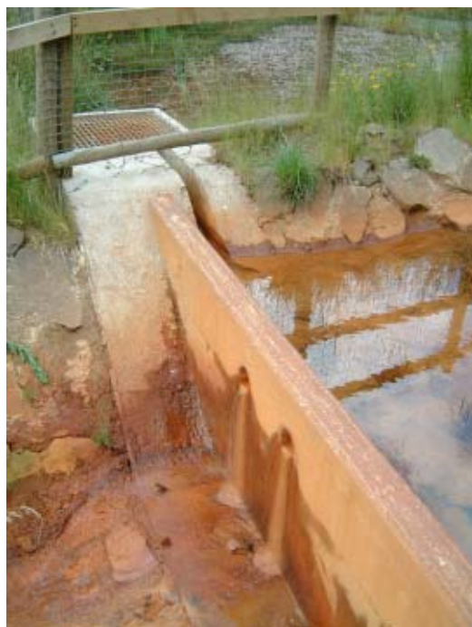
Figure 5.16.2. Diversion of part of stream flow from level B to wetland.
