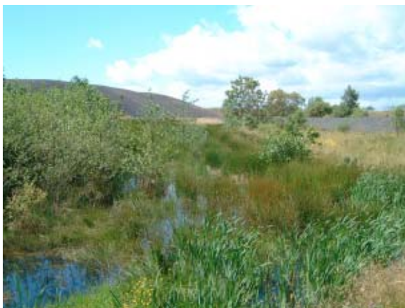
Figure 5.27.6. Wetland area incorporated as polishing mechanism into Polkemmet treatment scheme.
