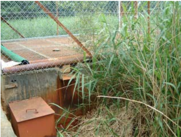
Figure 5.10.2. Holding tank, overflow to wetland and valve arrangement (in box) to allow water to be diverted to wetland when needed.
