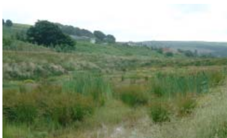
Figure 5.26.11. Gwenffrwd system SAPS. Note less ochre build-up on surface due to lack of minewater flow to this system for the period end 1998 to early 2001/.
