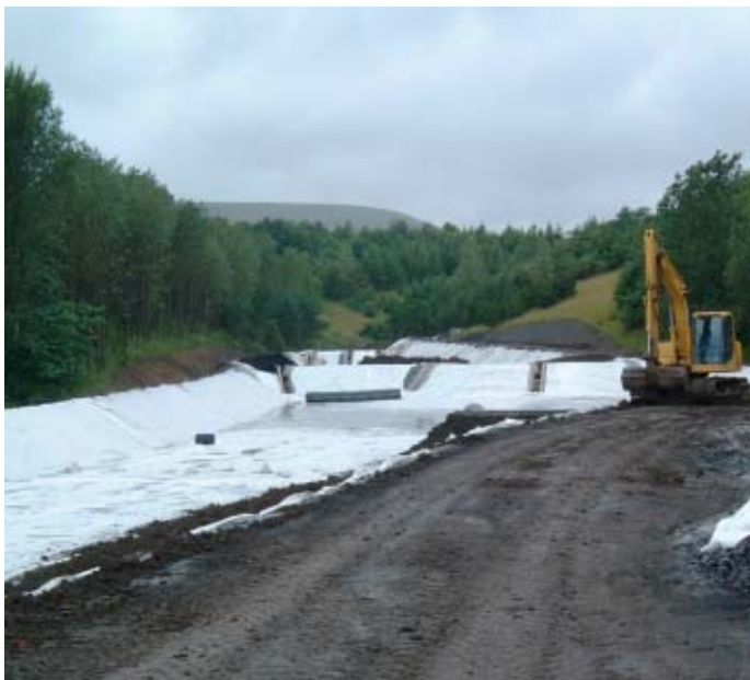
Figure 5.5.3. View of the reed bed construction, from the third cell looking ‘upstream’, showing how the scheme has been fitted into the narrow valley.
