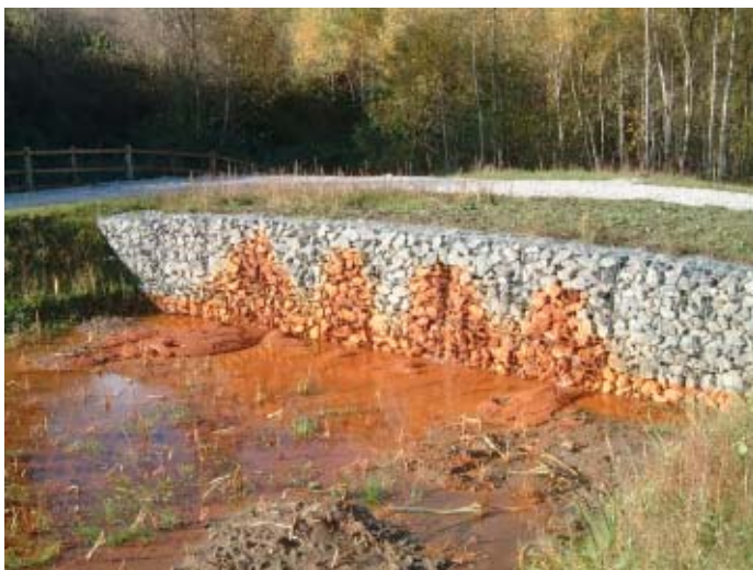
Figure 5.13.1. Gabion baskets at the inlet to the first wetland cell. Note the heavy ochre precipitation and poor plant growth.
