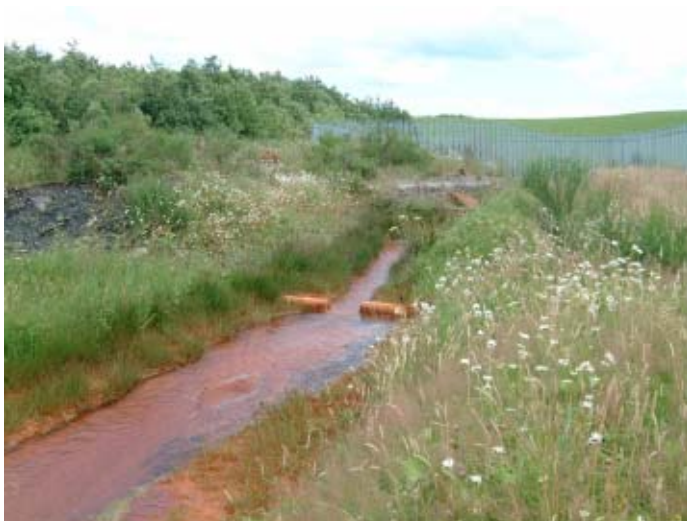
Figure 5.20.1. Minewater aeration cascade below issue point – the mineshaft is within the metal-fenced area.
