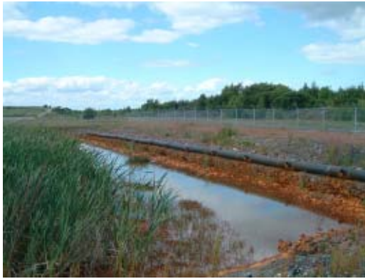
Figure 5.21.3. Reed bed cell, showing inlet pipe arrangement.
