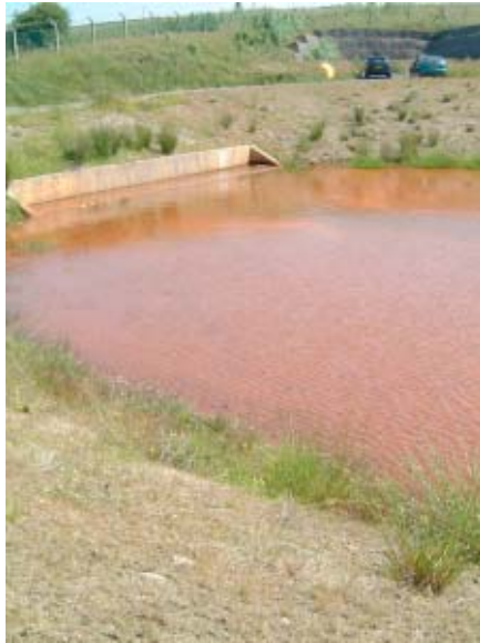
Figure 5.25.2. Inflow to first settling lagoon at Old Meadows, showing ochre build-up.
