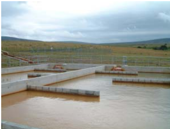
Figure 5.17.2. Settlement tanks at Kames – two tanks in parallel. The stepped aeration channel is to the left of the picture and the fenced area beyond the tanks is the location of the shaft.
