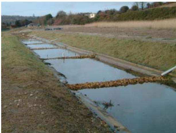
Figure 5.35.8. Rock filter, with anaerobic cell and aerobic cells to the right.
