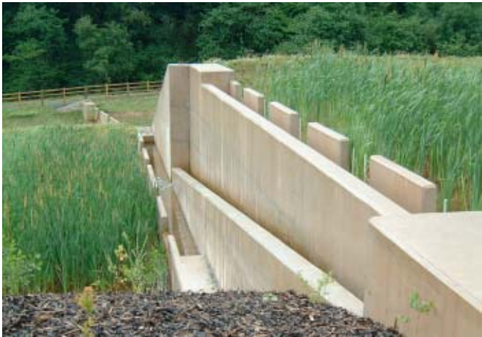
Figure 5.33.2. Concrete structure between consecutive cells at Taff Merthyr, showing change in height between cells.
