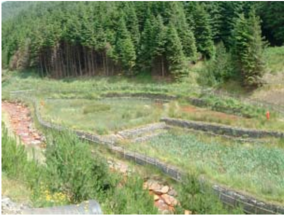
Figure 5.16.3. Wetland area – input from level B is near the red lifebuoy, outflow point is off to the right of the picture. Note ferruginous staining of river from upstream, diffuse sources.
