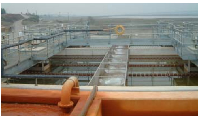
Figure 5.35.12. Clarifiers, at the final stage of treatment process – the central channel divides the two parallel streams of process water. The tailings dam is visible in the distance.
