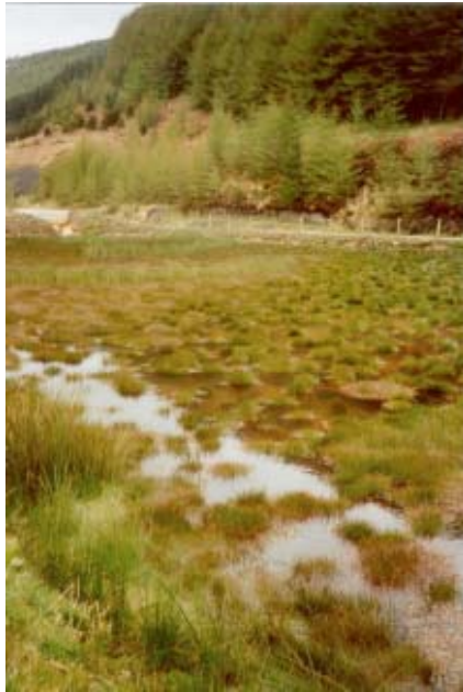
Figure 5.26.14. Garth Tonmawr – Cell 1, aerobic wetland and settlement lagoon, with natural colonisation.
