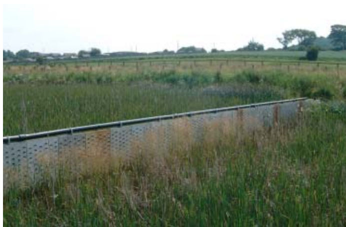
Figure 5.12.2. Dividing wall between cells, showing pipe along top of wall for raw minewater input, and small pipes through wall for between-cell flow.
