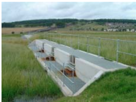
Figure 5.17.3. Between-cell re-aeration structure.
