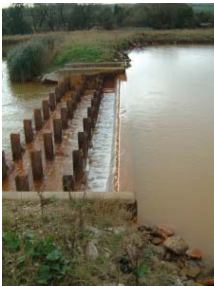
Figure 5.36.5. Weir structure and by-pass channel between first and second settlement lagoons – the vertical posts and wire mesh structures were incorporated to hold the filtration material, which is no longer necessary
