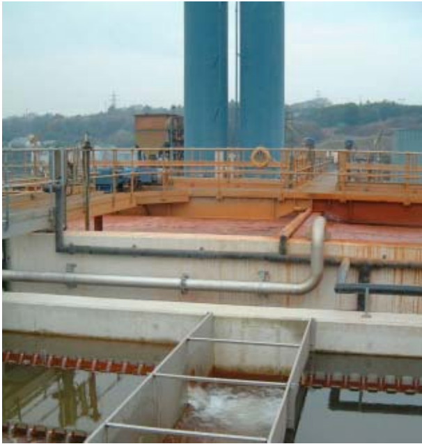
Figure 5.35.13. View of whole treatment plant, with lime storage silos in the background, sludge addition and lime addition/aeration tanks in the middle and clarifiers in the foreground.
