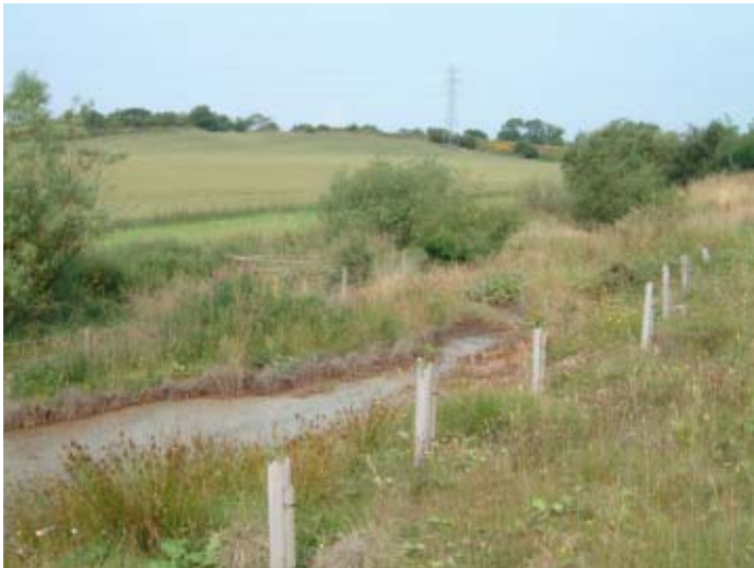
Figure 5.30.4. Drainage ditch along toe of spoil heap. The bushes mark the course of the burn and the bright green area beyond this is the site for river realignment and PRB construction.
