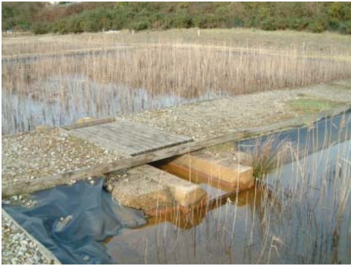
Figure 5.35.6. Concrete channel connecting consecutive aerobic cells.
