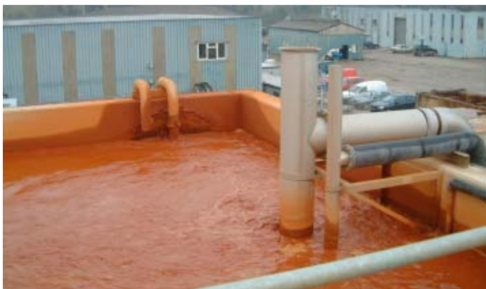
Figure 5.35.10. First tank of the treatment process, in which recirculated sludge is added.
