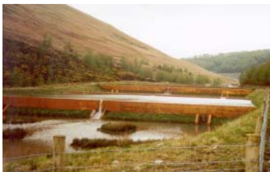
Figure 5.26.15. Garth Tonmawr – cell 5, aerobic wetland in the foreground, looking ‘upstream’. Flow from cell 4 to cell 5 is occurring over the top of the dividing wall, rather than through the pipes through the wall, at the top of the cascades, as intended
