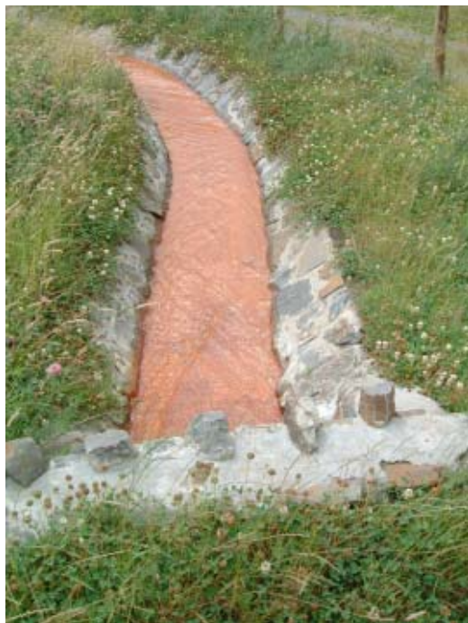
Figure 5.38.1. Channel taking pumped minewater from treatment plant to wetland (minewater is piped for most of the 1 km distance, with an open channel taking part of the water to the one of the wetland cells).
