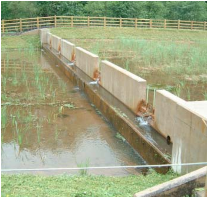
Figure 5.33.3. Concrete structure between cells.
