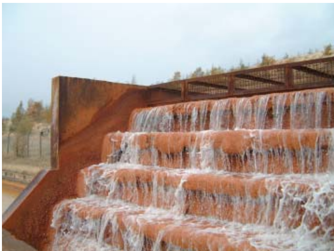
Figure 5.36.2. Aeration cascade at inlet to second settlement tank – the overall height of the cascade structure is about 2 m.
