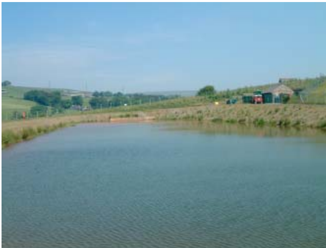
Figure 5.25.3. View of first settling lagoon, with the active dosing plant housed in the building on the right.
