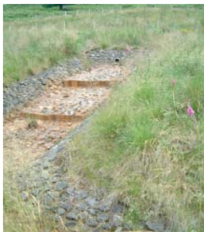
Figure 5.26.10. Gwenffrwd system ochre accretion terrace.
