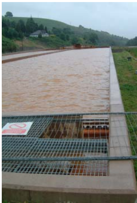
Figure 5.33.1. Sludge settling tanks at Taff Merthyr.
