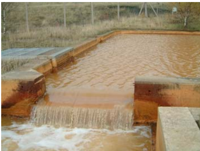
Figure 5.36.3. Outflow from third settlement tank.
