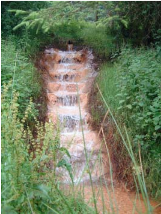
Figure 5.19.1. The inflow cascade to the Mains of Blairingone treatment wetland.
