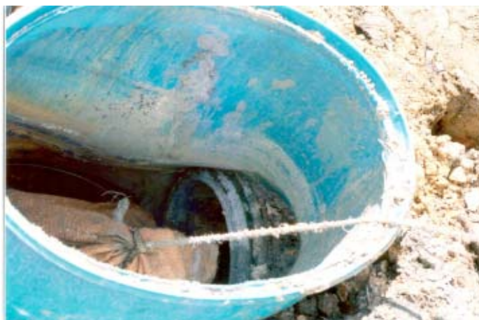
Figure 5.22.3. Dosing system for sodium carbonate.
