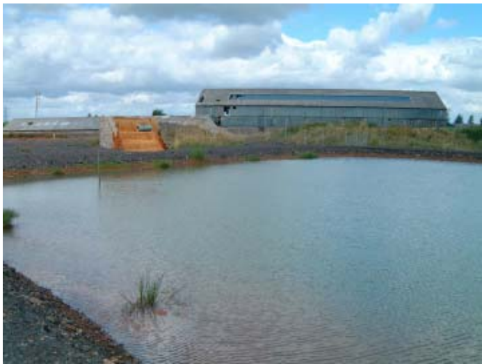
Figure 5.27.4. Secondary lagoon of current treatment system (this was the main lagoon of the original treatment system – note disused aeration cascade).
