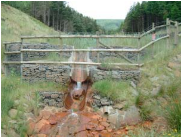
Figure 5.16.4. Outflow from reed bed 3 – by-pass flow from level B is to the right of the picture, the re-aligned river is to the left.
