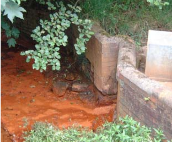
Figure 5.10.1. Discharge point from minewater holding tank to the burn.
