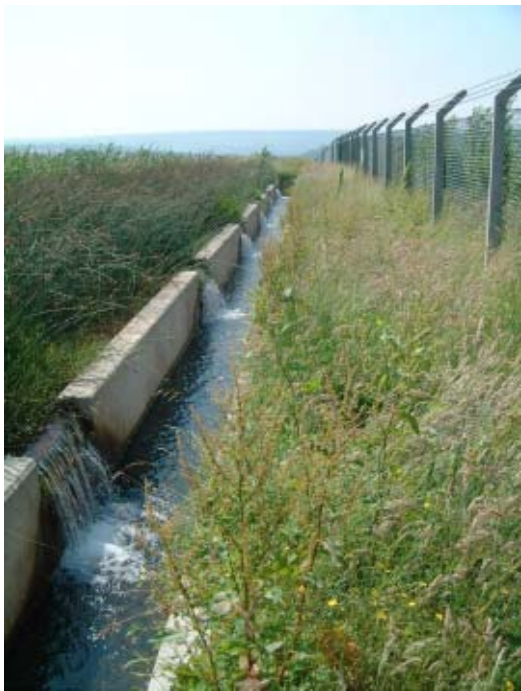
Figure 5.25.5. Outflow from reed bed cell.
