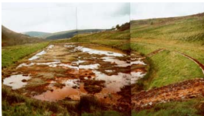
Figure 5.26.8. Whitworth A SAPS, showing distribution channel and ochre build-up on the surface.
