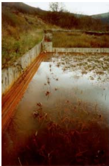
Figure 5.26.4. Whitworth 1 wetland, showing flow distribution channels for cells (the water level in the cell in the foreground is higher than it should be).
