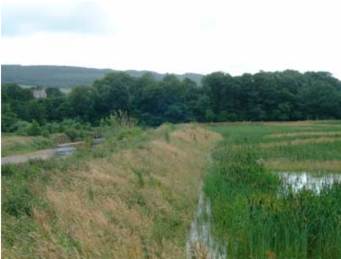
Figure 5.38.3. Earth bund separating wetland (right) from the river (left).
