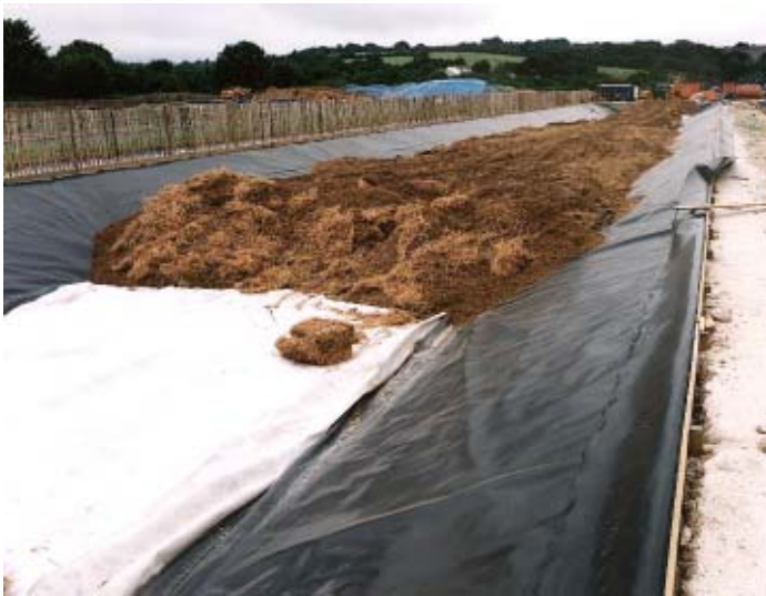
Figure 5.35.7. Anaerobic cell during its construction showing organic material.
