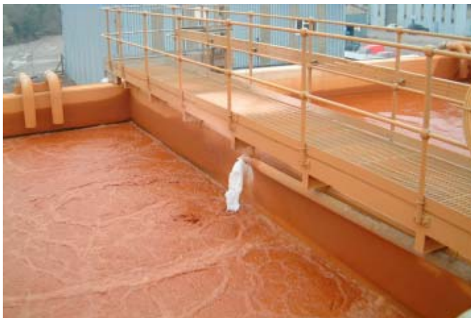
Figure 5.35.11. Second tank, in which lime slurry is added and aeration carried out.
