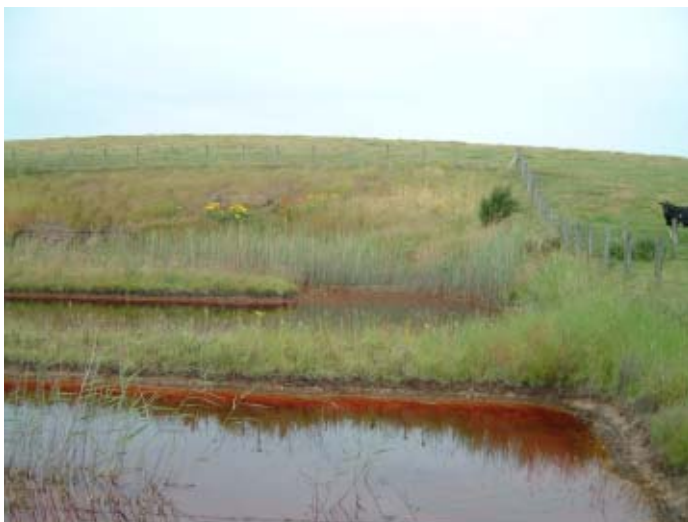
Figure 5.15.2. The wetland cell at Gilmerton, looking towards the inflow and showing the reclaimed bing behind the wetland and the bunds extending across the width of the cell.
