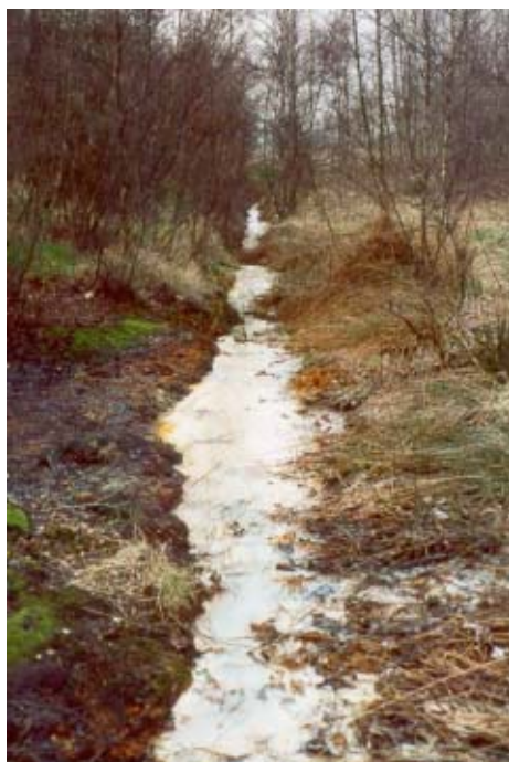
Figure 5.11.2. Drainage ditch between trial reed bed and reed bed 1; note Al precipitates. Spoil heap is to the left of this photograph (photo courtesy of John Hine).
