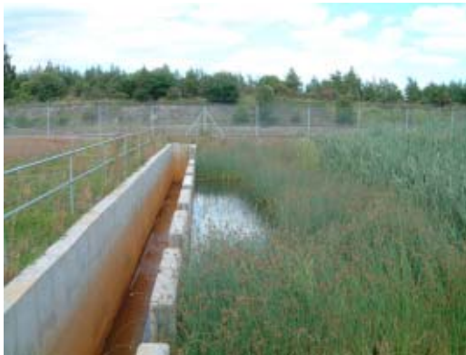
Figure 5.21.4. Outlet from reed bed cell.
