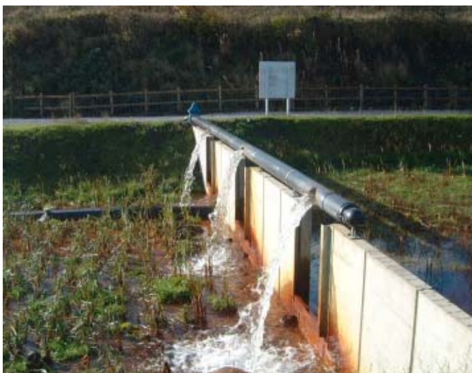
Figure 5.13.2. Inlet cascade to second wetland cell, being used to by-pass the first cell.
