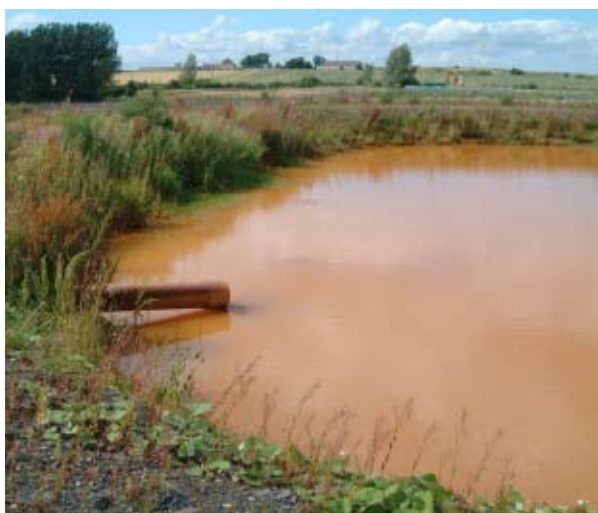
Figure 5.21.2. Settling lagoon, showing inlet pipe. The fence around the pumping station and shaft area can be seen in the middle distance, beyond the lagoon.
