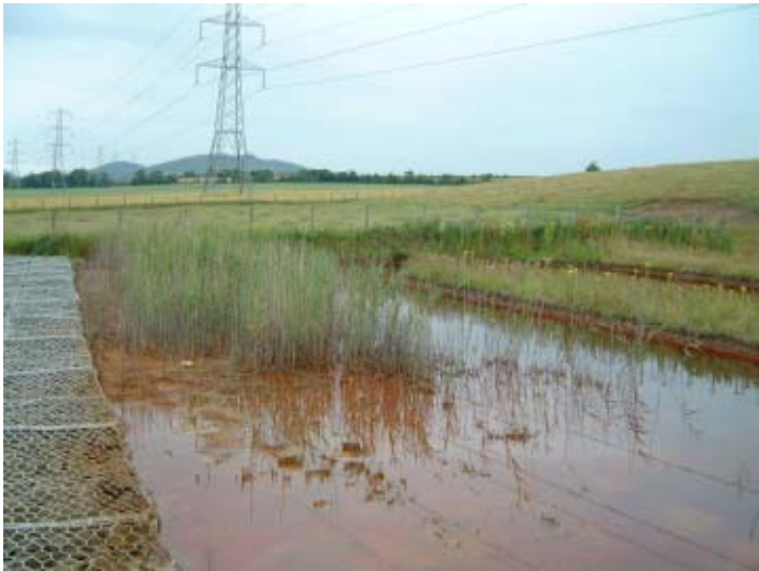
Figure 5.15.3. Gabion baskets at the outflow of the wetland cell.
