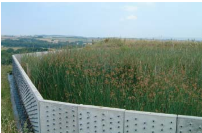
Figure 5.12.3. Outlet from the Edmondsley constructed wetland.
