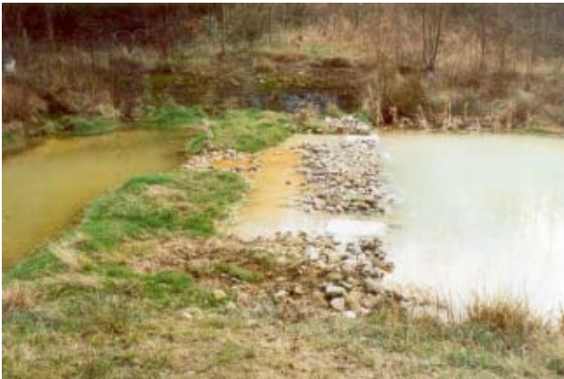
Figure 5.11.4. Settlement lagoon prior to discharge to reed bed 2. Sodium carbonate is added; note bags of this on the dividing bund, and also note precipitation of Al following this addition (flow is from left to right) (photo courtesy of John Hine).
