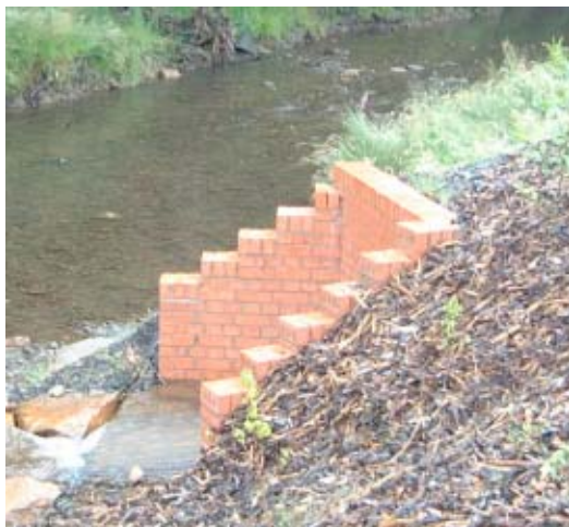
Figure 5.33.4. Outfall from Taff Merthyr treatment system to the river.
