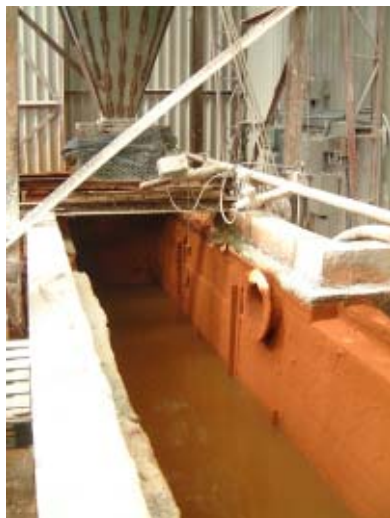
Figure 5.21.1. Lime dosing system, showing dosing tank and screw hopper for introduction of lime. The pipe in the wall of the tank is the outflow to the settling tanks.
