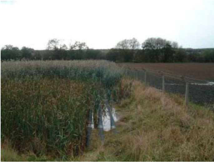
Figure 5.36.7. Plastic pipes at inlet to wetland area.
