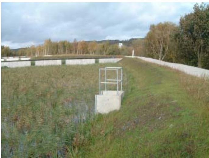
Figure 5.13.3. One of the three outlet structures from fourth wetland cell.
