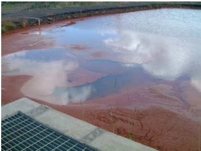
Figure 5.27.3. Inflow zone to primary settlement lagoon, showing flow-splitting chamber and ochre accumulation.
