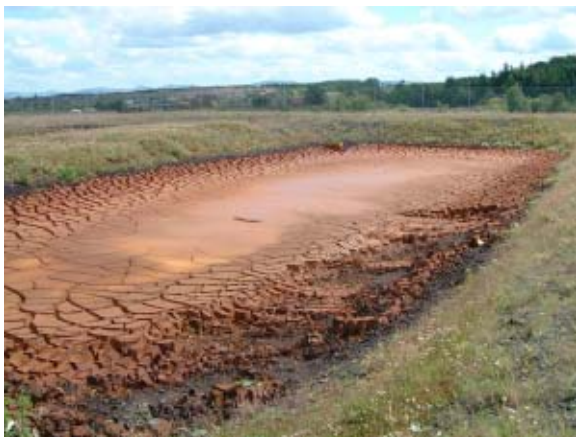
Figure 5.27.5. Sludge-drying/storage lagoon (which was one of the secondary lagoons of the original system).
