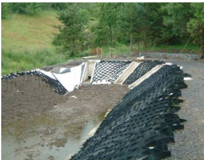
Figure 5.5.2. First reed bed cell during construction, showing inlet structures, lining material, bank stabilisation material and topsoiling in process.
