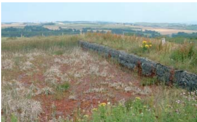
Figure 5.12.1. Inlet to first wetland cell, showing gabion baskets through which flow occurs. Note poor Typha growth and ochre accumulation. The Scirpus at the far end of the wall, middle left of the photograph, appear to be more healthy than the Typha .
